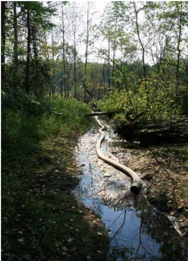
Beavers responded by chewing the pipe in half! A full scale assault resulted with men invading the ponds in waders, clearing bunged baffles, patching the severed “O” drain and wrapping it with the ever popular chicken wire. The team felt the campaign had been effective and regrouped over coffee (in damp, muddy gear) declaring a modest victory.
